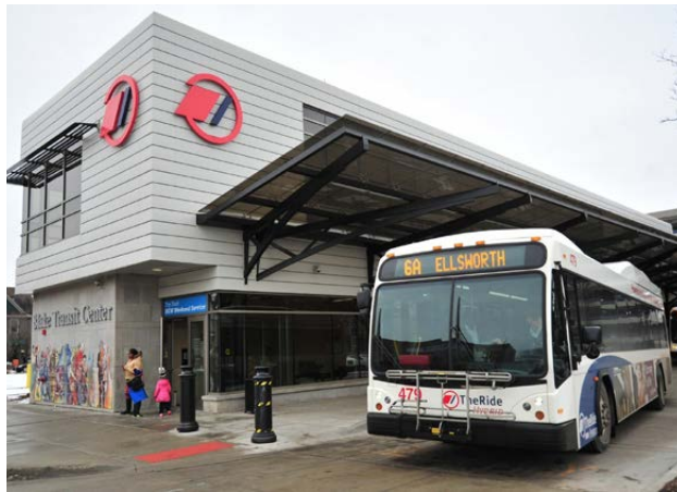
TheRide consists of a comprehensive network of bus service providing safe, reliable connections throughout the city.
