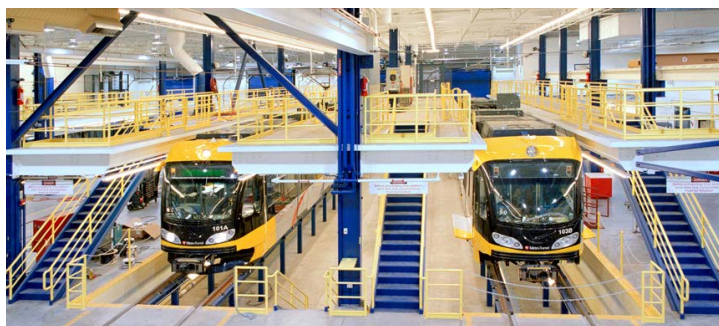
Minneapolis LRT Maintenance Facility
