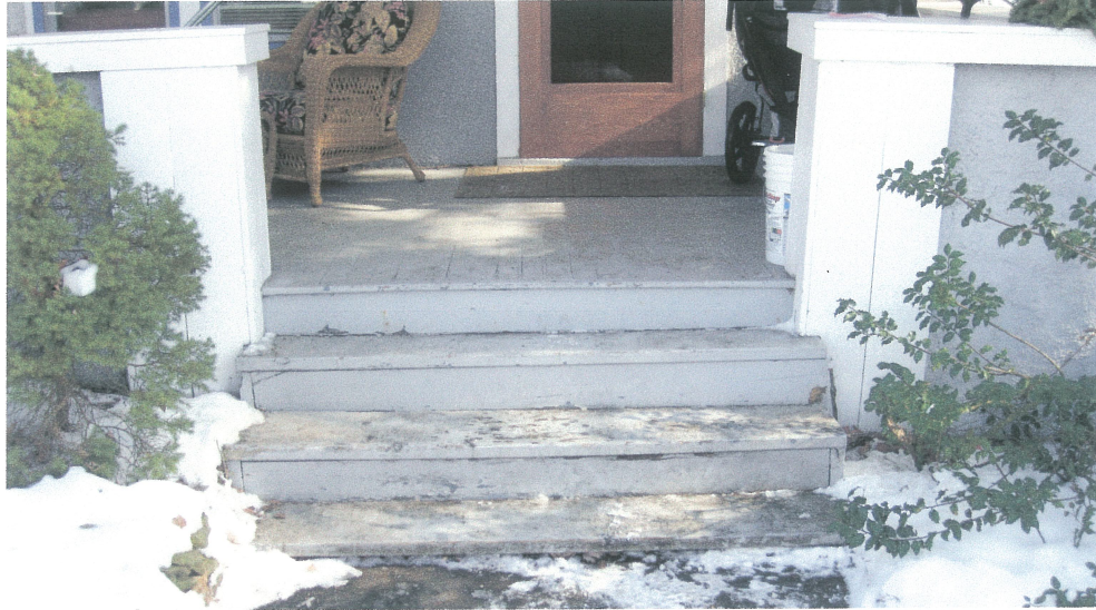
Steps on Front Porch to be replaced
