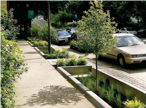
Example of Stormwater Parkway Planters
