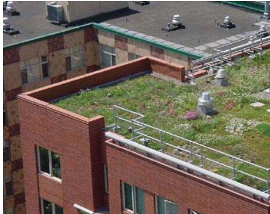
Example of Vegetative Roof
