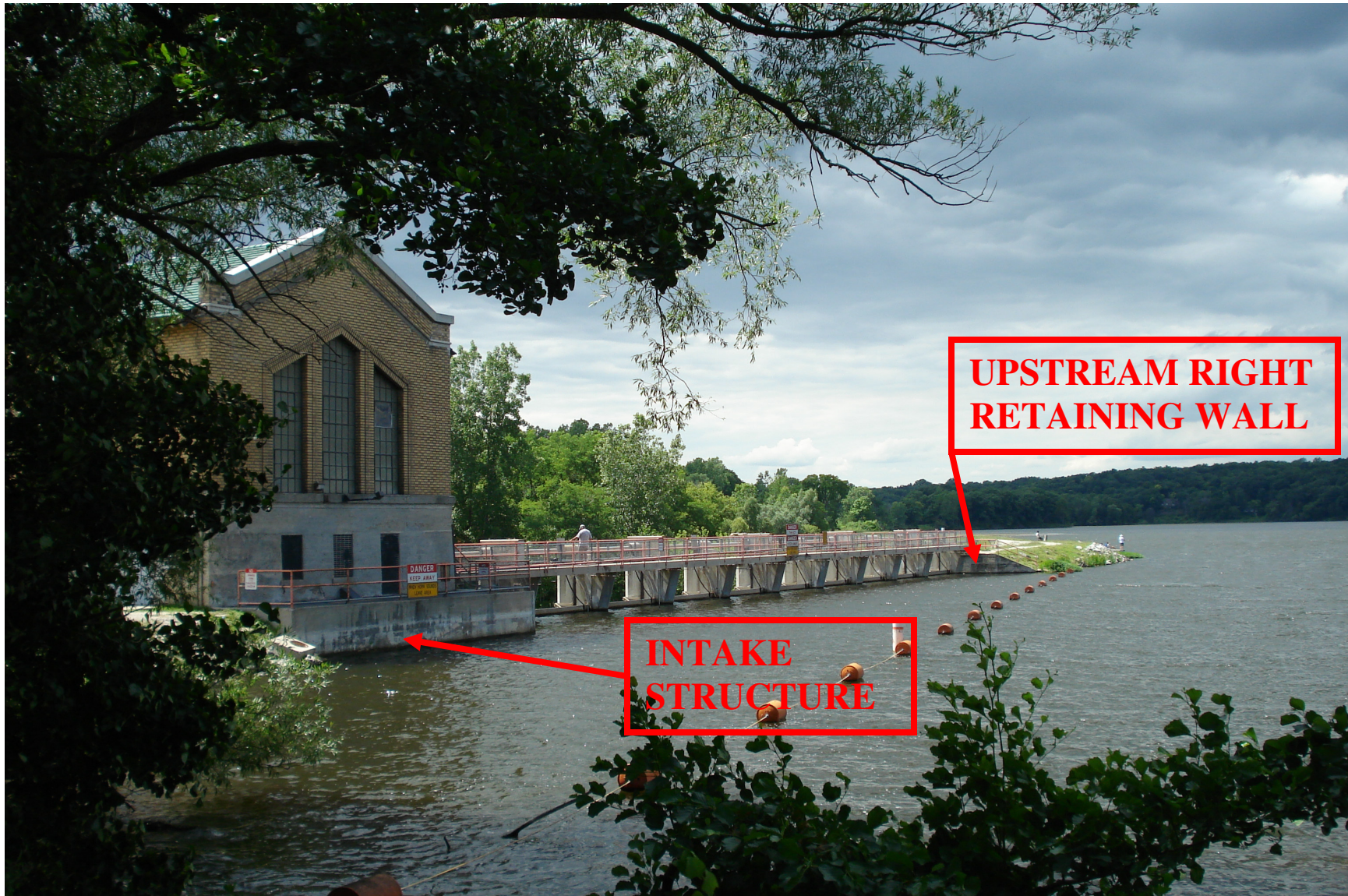
Intake Structure – Cores shall be taken into the vertical faces of the intake structure just above the water line.
