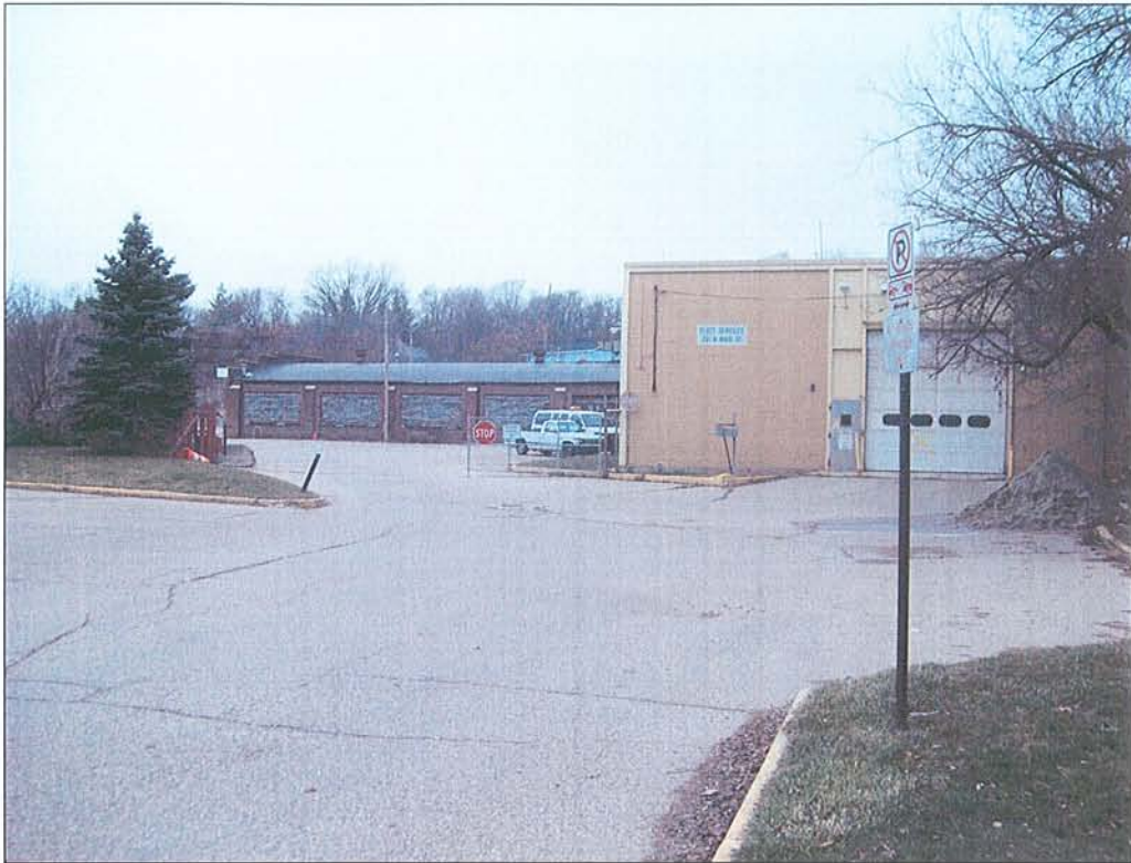
PHOTO NO. 11: Former City Garage, adjoining the Property to the west.
