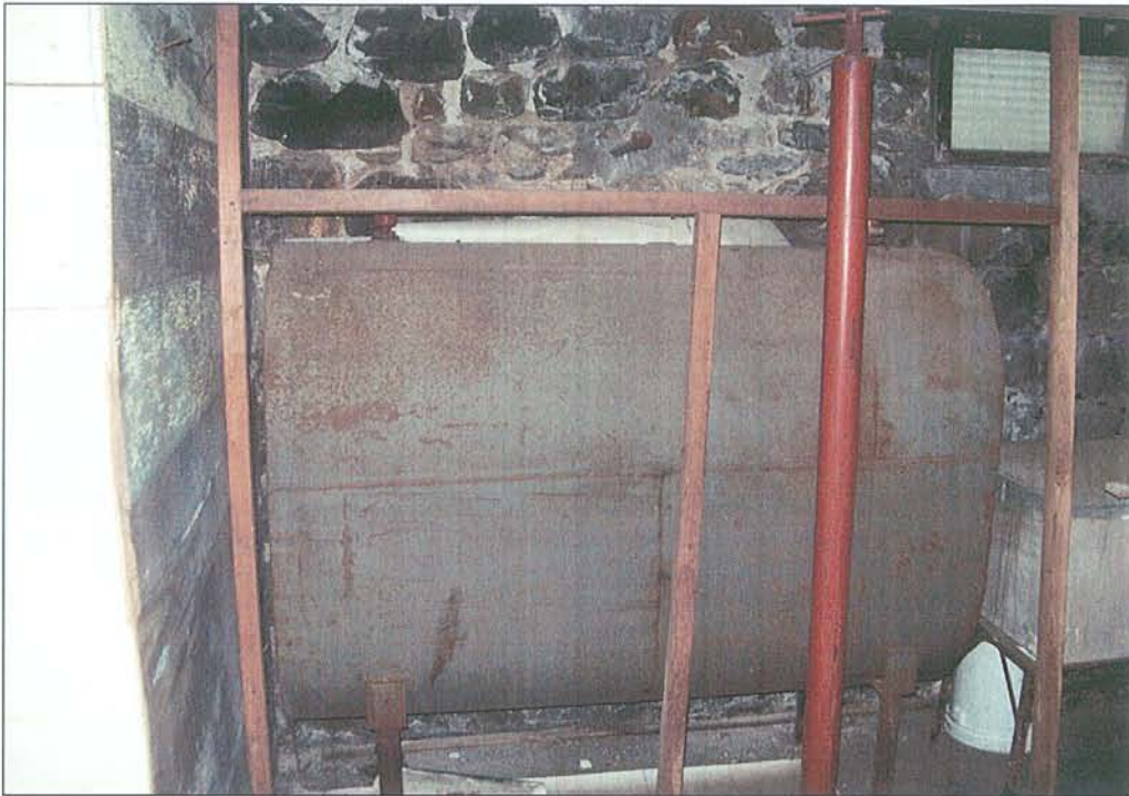
PHOTO NO. 5: A 250-gallon aboveground storage tank, located in the basement of 626 North Main Street.
