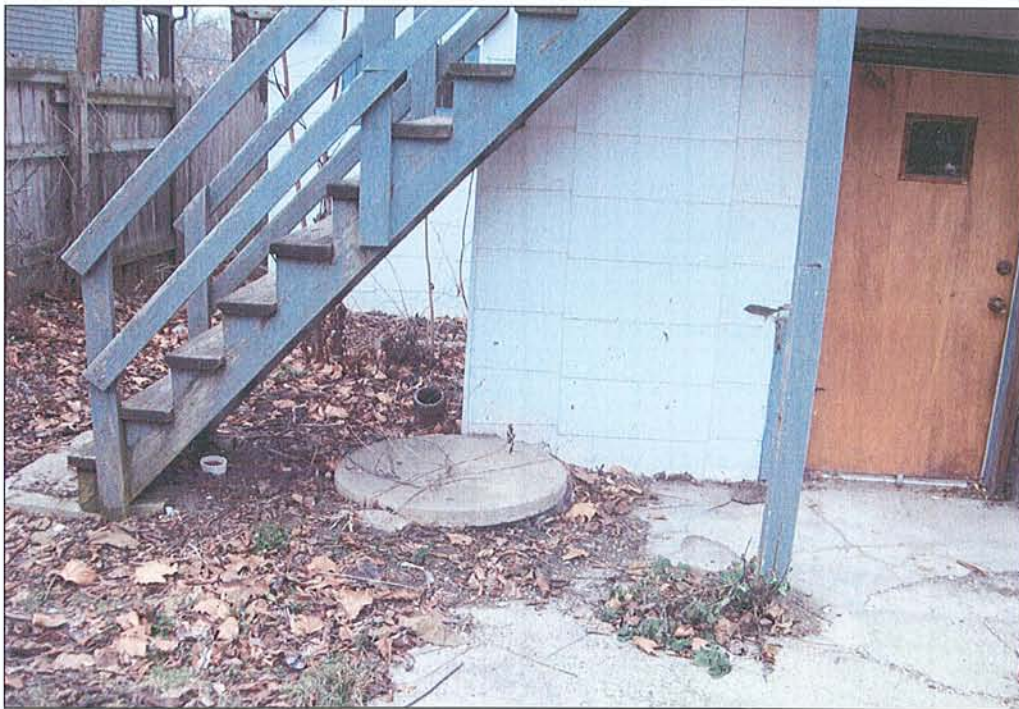
PHOTO NO. 4: A cistern, located on the southwest corner of residential dwellings (626 North Main Street).
