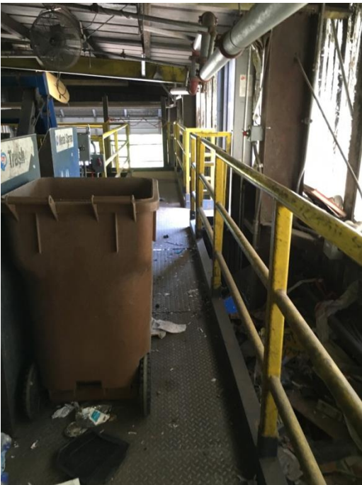
Blocked fire egress.
