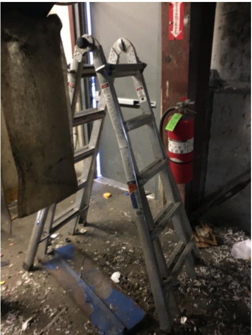
Blocked emergency exit and fire extinguisher
