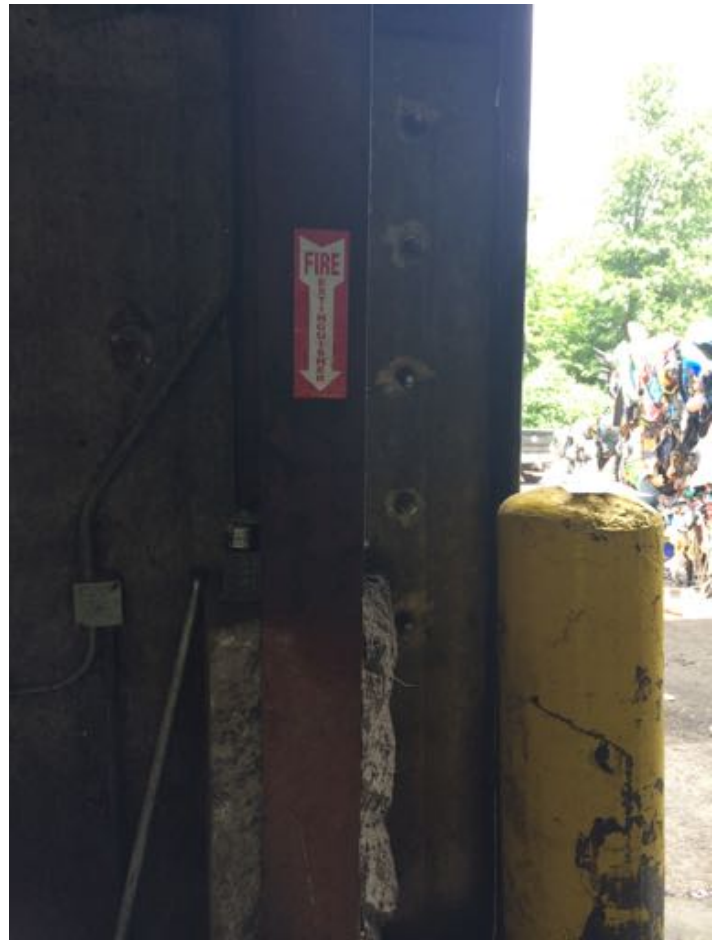
All: Fire extinguishers missing or inaccessible
