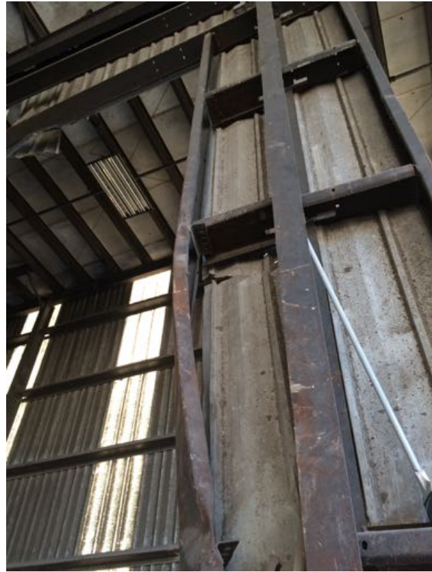
Top: Structural damage – struck by equipment
