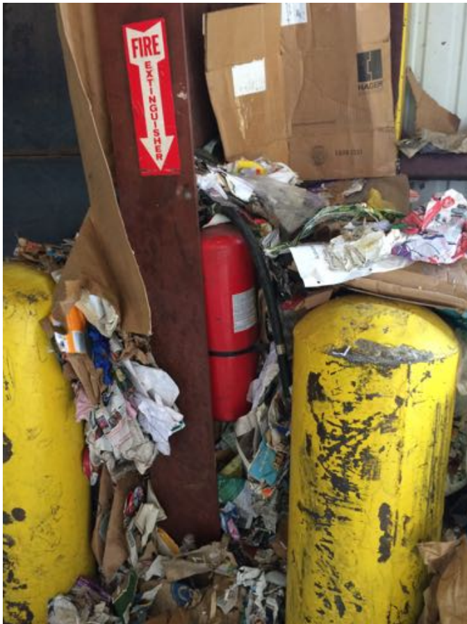
All: Fire extinguishers missing or inaccessible
