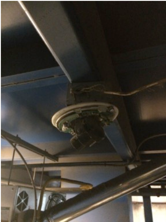
All: Exposed wiring Bottom right: dust/debris build-up
