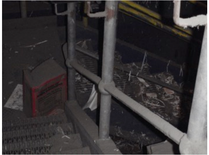
Top left: wiring under conveyer with debris over/under/on/around wire
