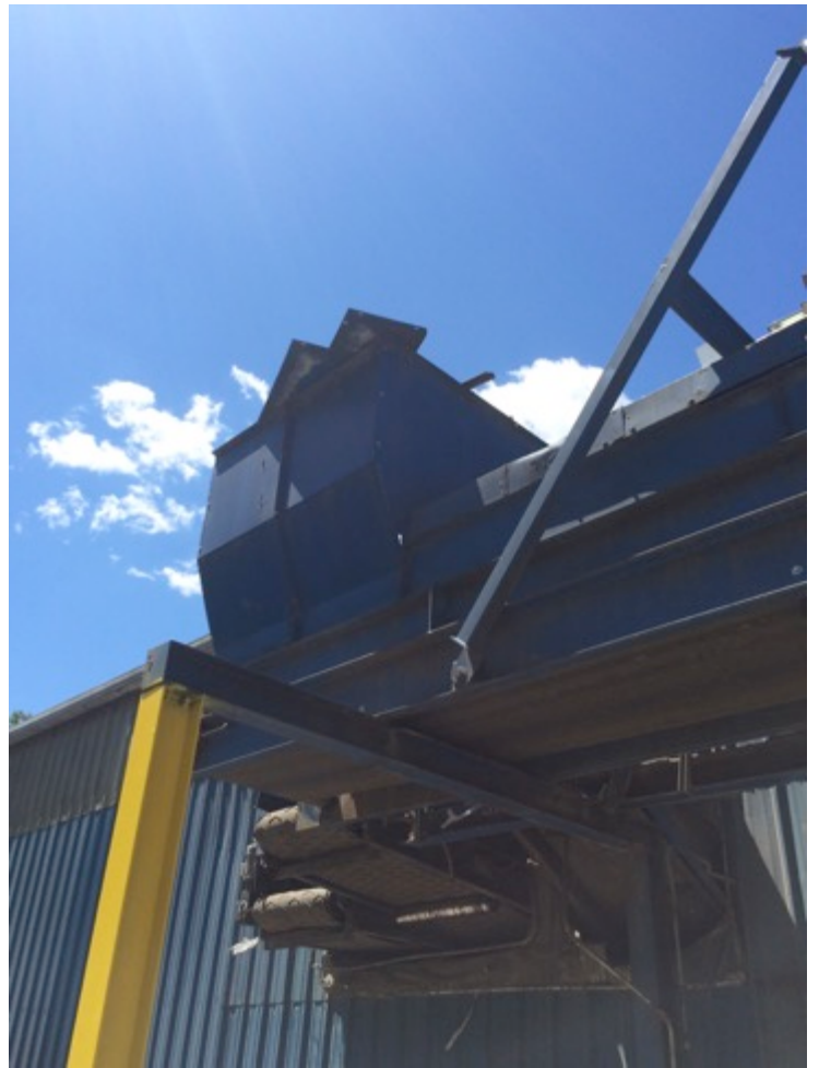
Top left: exposed wiring
