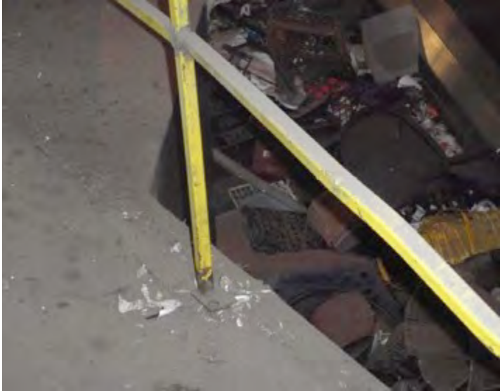
Hand rail needs repair in two spots
