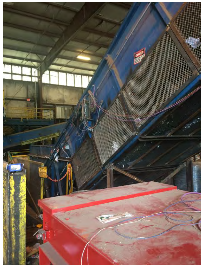
Lots of uncapped wires, potential shock hazard. (work in progress)
