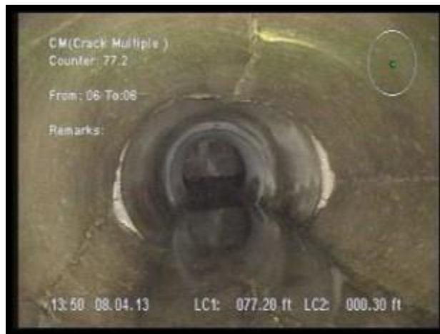
Figure II-9: Minor Sewer Cracks
