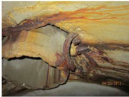
Photo 22 branch "A" station 14+32: 12" concrete pipe (bulk headed)
