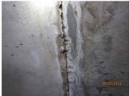
Photo 17 branch "A" station 10+08: pipe joint, minor spalling
