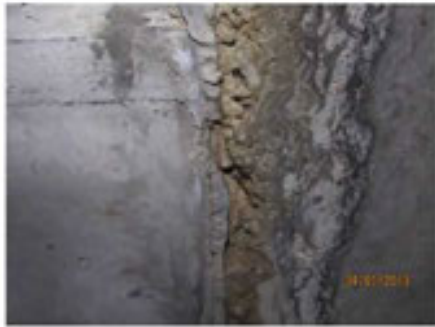
Photo 13 branch "A" station B+44: pipe joint, minor spalling
