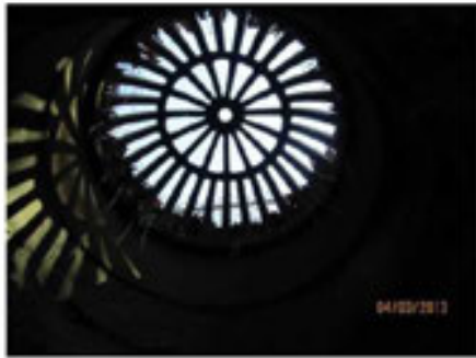
Photo 19 branch "A" station 11+66 (R5): beehive inlet
