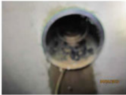
Photo 46 branch "B" station 3+50: 6" PVC pipe
