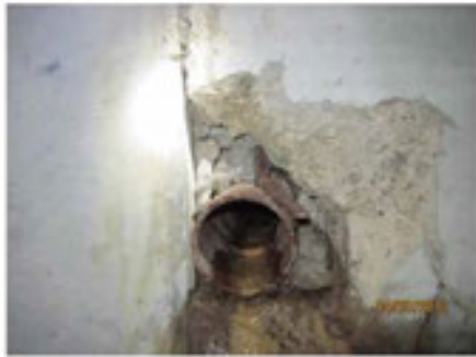
Photo 16 branch "A" station 9+50: 4" cast iron pipe
