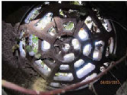
Photo 5 branch "A" station 4+80 (R3): beehive inlet
