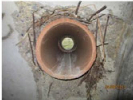
Photo 35 branch "A" station 25+34: 12" clay pipe
