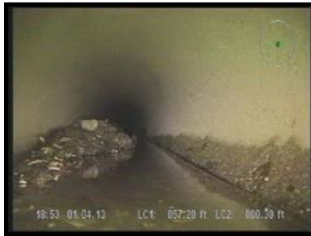
Figure II-8: Sewer Blockage
