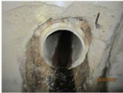
Photo 10 branch "A" station 7+88: 12" concrete pipe
