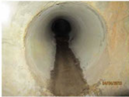
Photo 31 branch "A" station 21+71: 15" concrete pipe
