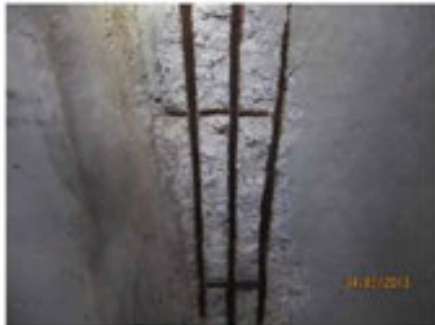
Photo 11 branch "A" station 8+04 pipe joint, minor spalling
