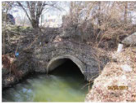
Photo 1 branch "A" station 1+00(R1): 72" pipe outlet
