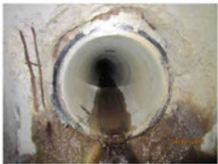
Photo 6 branch "A" station 5+58: 15" concrete pipe
