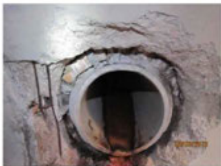
Photo 15 branch "A" station B+95: 15" concrete pipe
