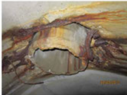
Photo 23 branch "A" station 14+32: 12" concrete pipe (bulk headed)
