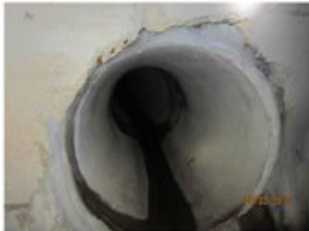
Photo 20 branch "A" station 13+83: 42" concrete pipe
