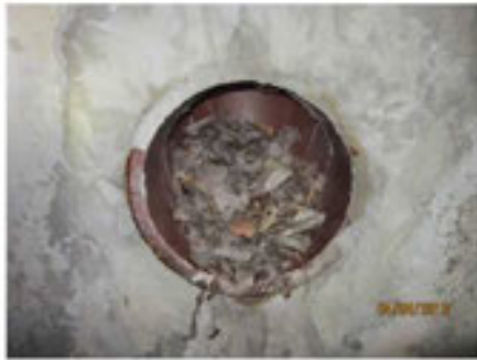
Photo 28 branch "A" station 20+15: 12" clay pipe
