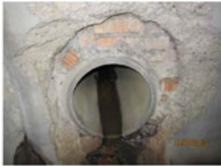
Photo 4 branch "A" station 3+85: 15" concrete pipe
