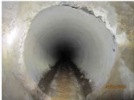
Photo 44 branch "B" station 3+40: 12" concrete pipe
