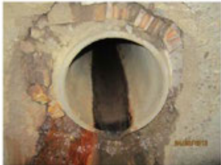
Photo 14 branch "A" station B+90: 15" concrete pipe
