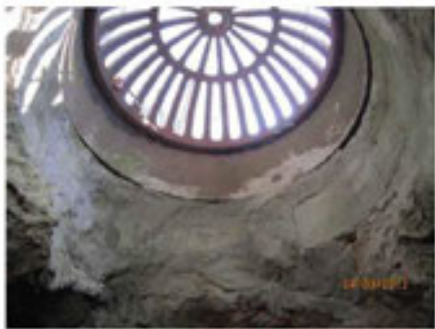
Photo 24 branch "A" station 16+42 (R6): beehive inlet
