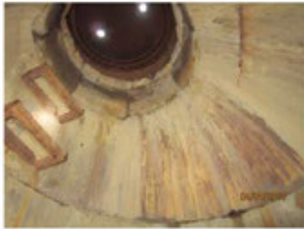
Photo 43 branch "B" station 3+40 (RS): precast manhole structure
