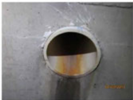
Photo 12 branch "A" station 8+22: 4" PVC pipe
