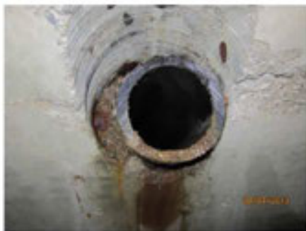
Photo 51 branch "B" station 7+10: 4" PVC pipe
