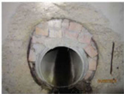
Photo 18 branch "A" station 10+75: 12" concrete pipe
