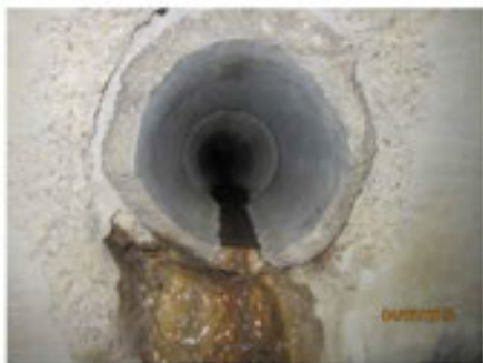
Photo 21 branch "A" station 13+95: 18" concrete pipe
