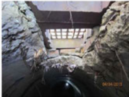
Photo 47 branch "B" station 5+25: flat grate inlet
