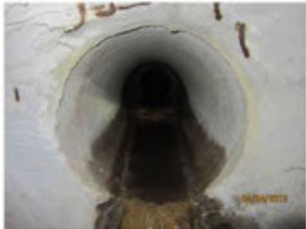
Photo 38 branch "A" station 28+91: 15" concrete pipe
