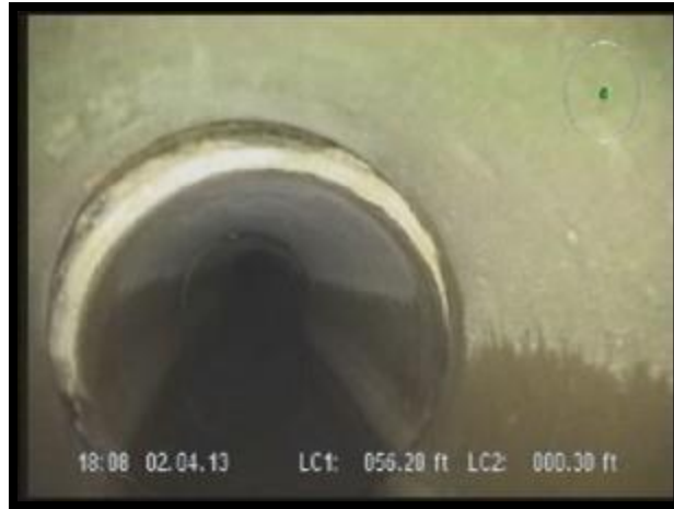
Figure II-10: Broken Pipes
