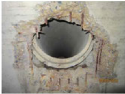
Photo 34 branch "A" station 24+03: 12" concrete pipe
