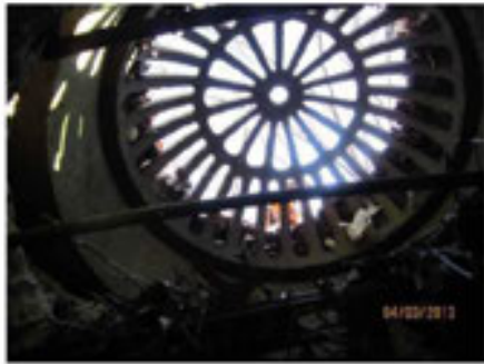
Photo 25 branch "A" station 17+34; beehive inlet
