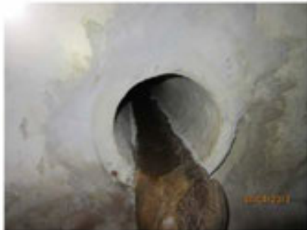
Photo 29 branch "A" station 21+70: 12" concrete pipe
