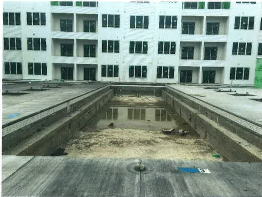
Vinyl siding installation and poured pool deck.
