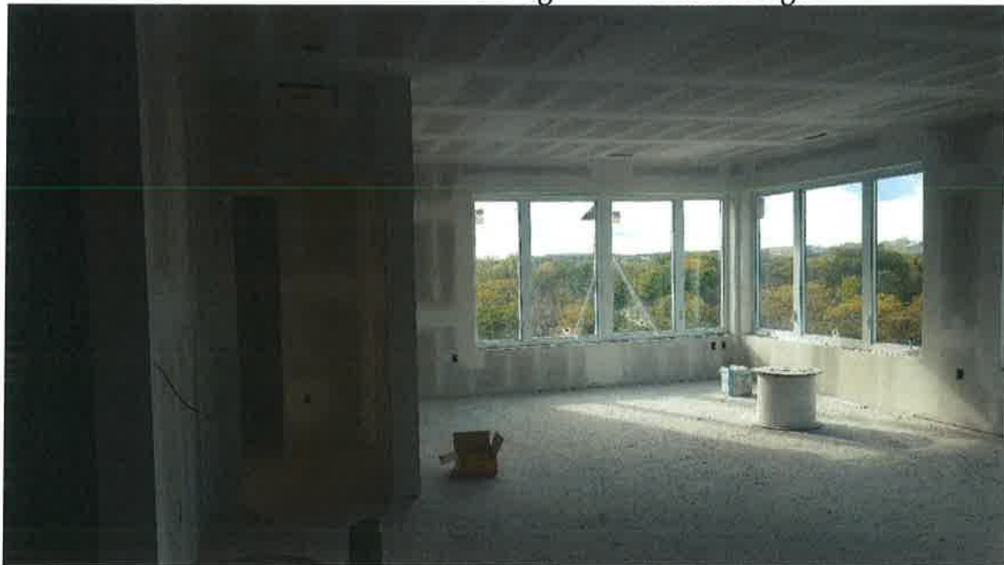
Drywall installation in 4 th floor unit.
