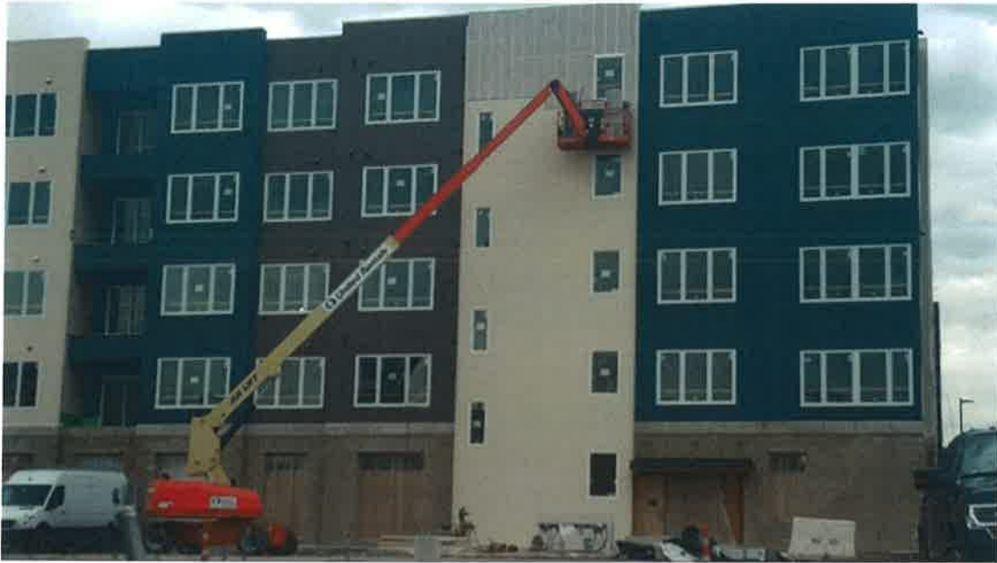
Fiber cement siding installation.
