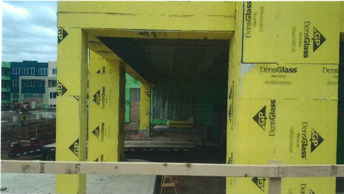
Installation of the exterior framing in the drive-through areas.
