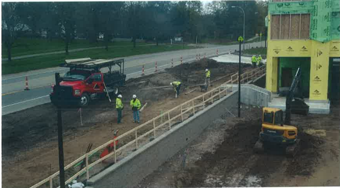
Right of way work and sidewalk preparation.
