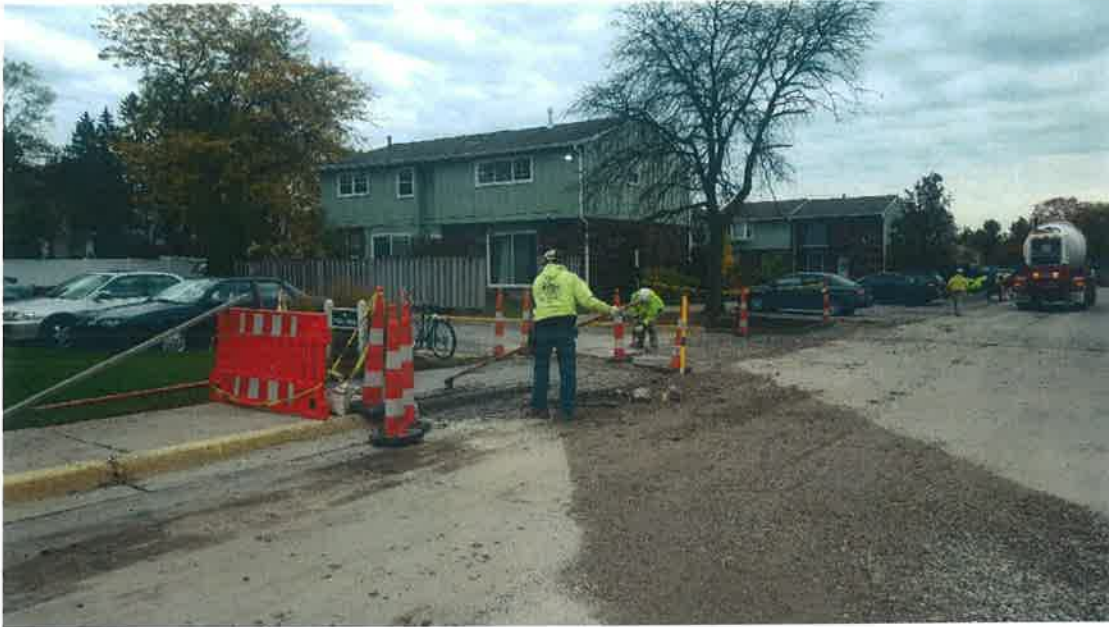
Concrete work at Georgetown Condominiums.
