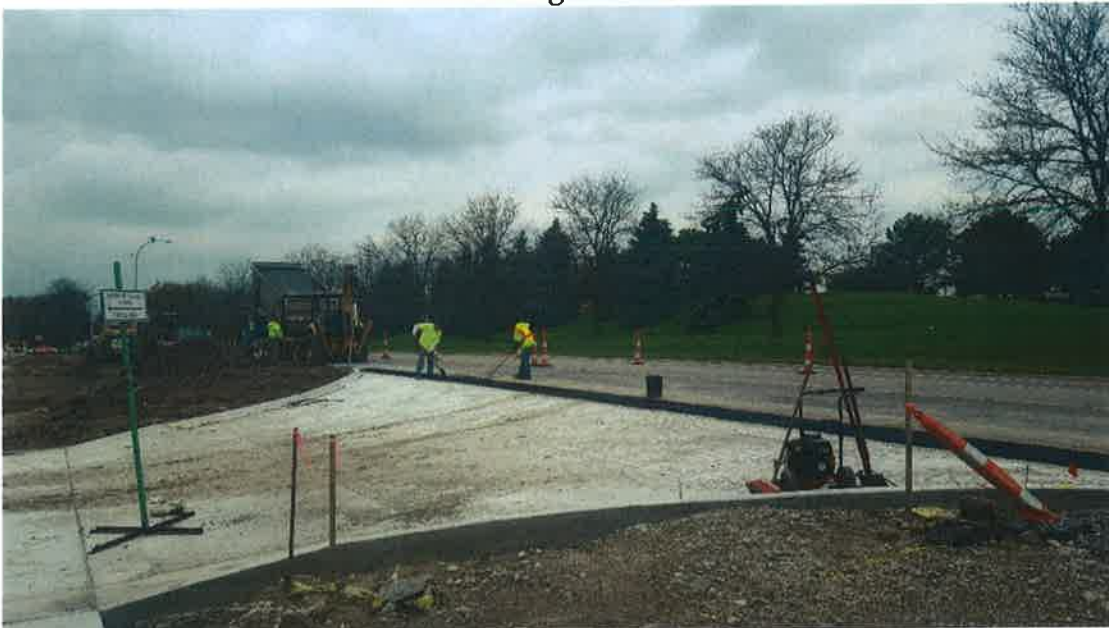
Packard Street approach installation in process.
