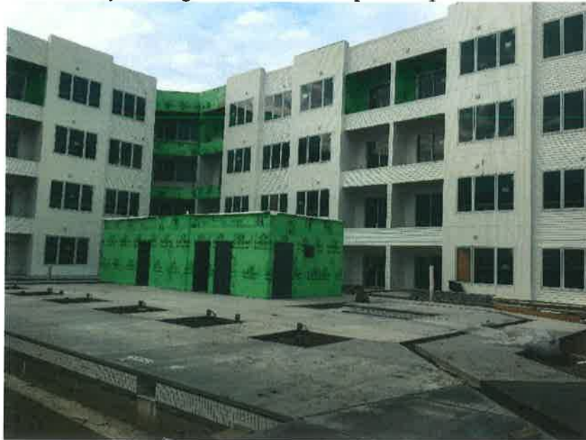
Vinyl siding installation and poured pool deck.
