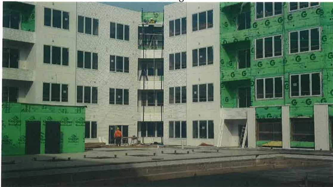
Vinyl siding installation.
