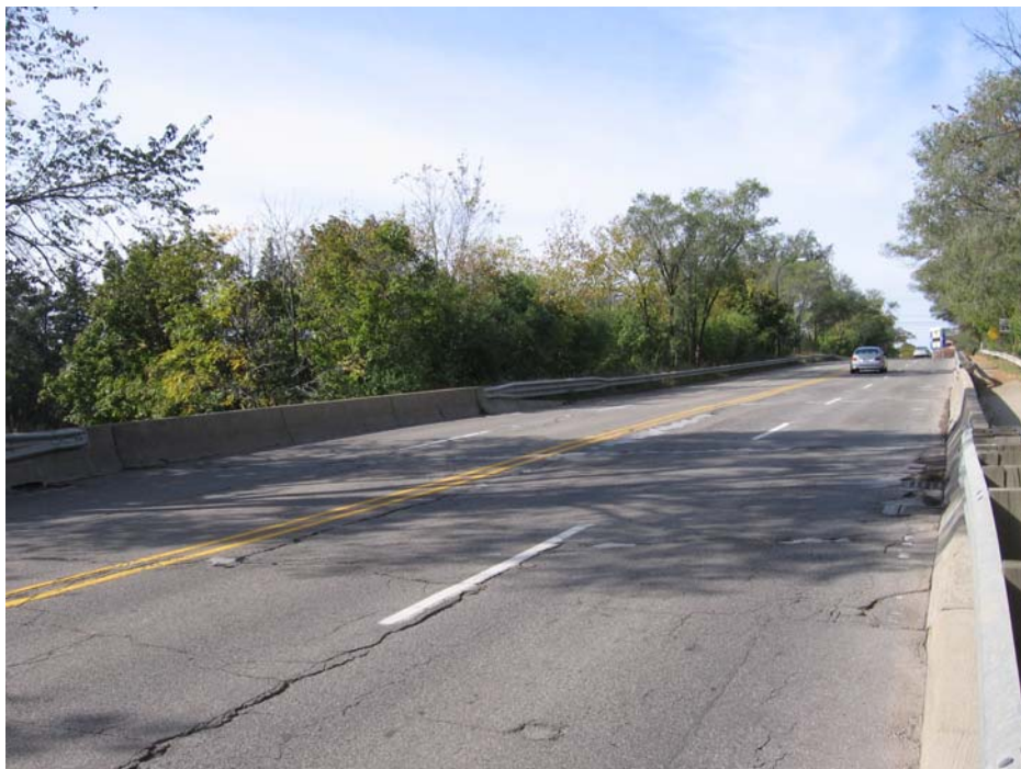
Photo 2: Stadium Boulevard over State Street looking West.
