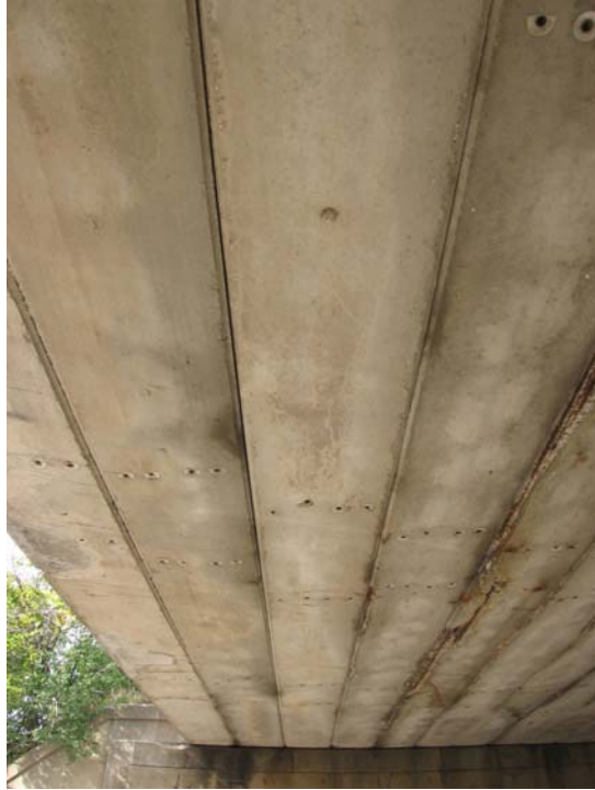
Photo 11: Picture showing west side of bottom of beams with spalled concrete and exposed reinforcing strands on south side of bridge.
