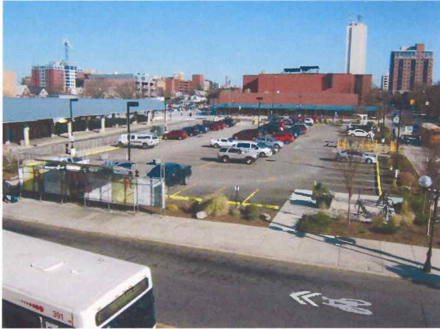
Elevated view of the subject looking east
