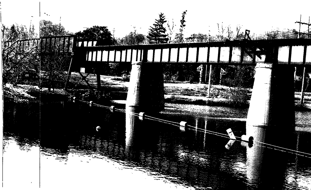
Photo 6: Right earth embankment and upstream bank. Float and cable system can also be seen. Nov. '92
