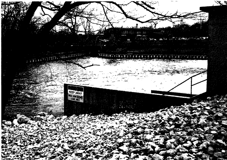
Photo 5: Rip-rap along downstream face of left embankment. Steel pilings along right downstream bank can be seen across spillway. Nov. '92
