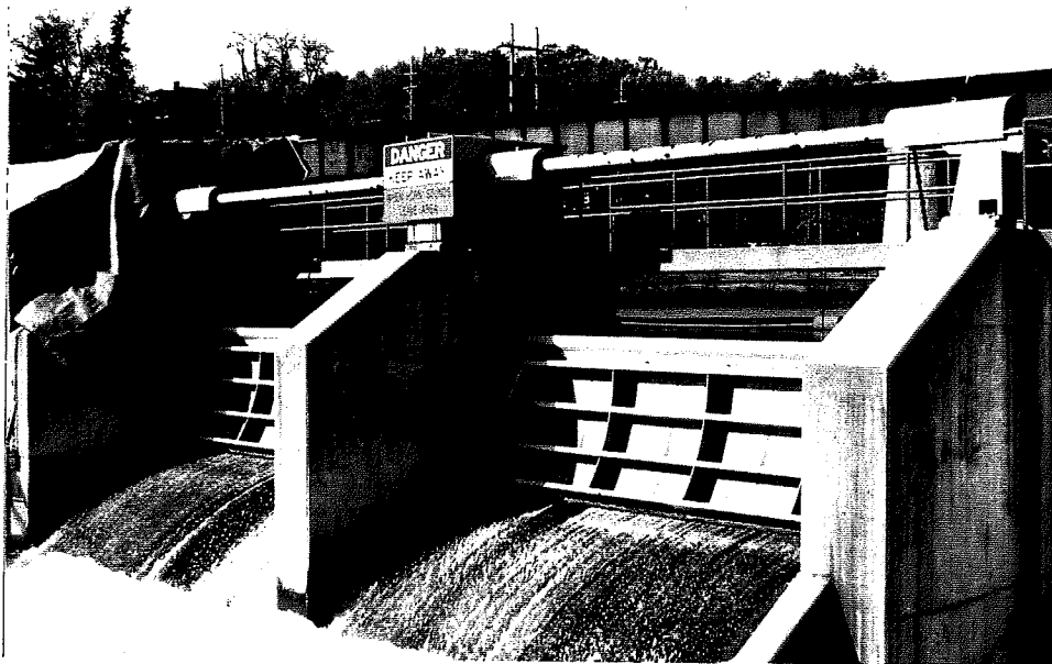
Photo 2: Two spillway bays with radial steel gates in operation. Nov. '92
