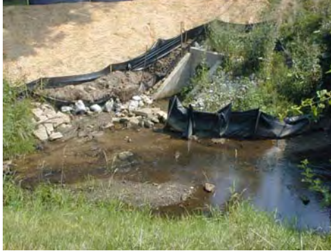
Road work is another source of soil erosion to the Mill Creek system, such as along this stretch of Letts Creek. Photo: HRWC
