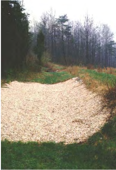
Infiltration trench. Photo: Center for Watershed Protection
