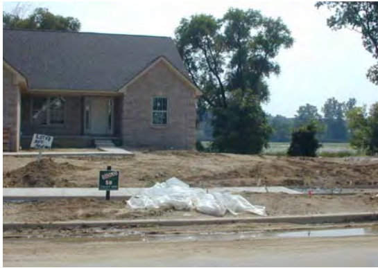
New development along lakeshores, in this case along Pierce Lake, often increases the amount of nonpoint sources of pollution in the waterbody. Photo: HRWC
