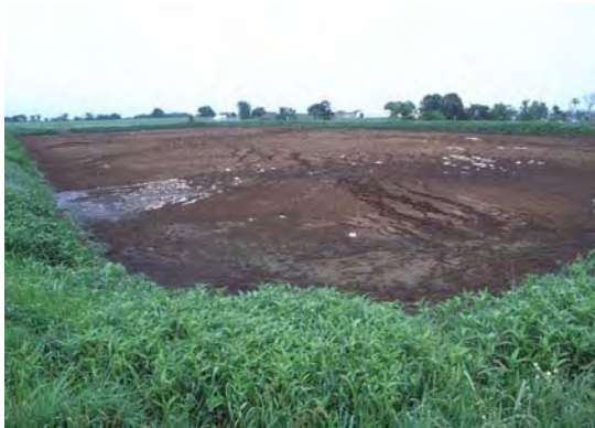
Waste storage facility. Photo: Washtenaw Co. Conservation District
