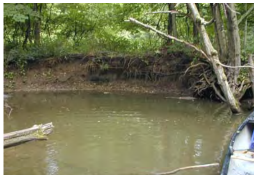
Evidence of scouring flows is seen along the mainstem near Sager Road in the form of these incised banks. Photo: HRWC
