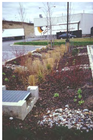
Bioretention System. Photo: Center for Watershed Protection
