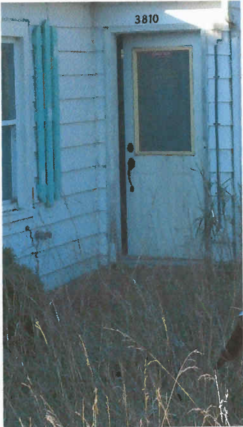
Open doors & siding issues
