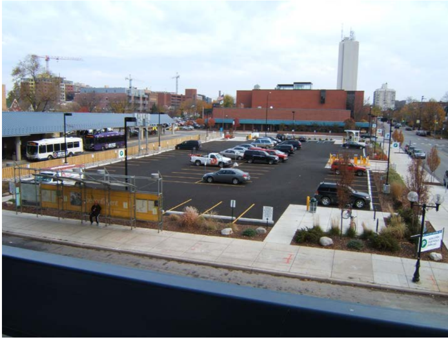
Elevated view of the subject looking east
