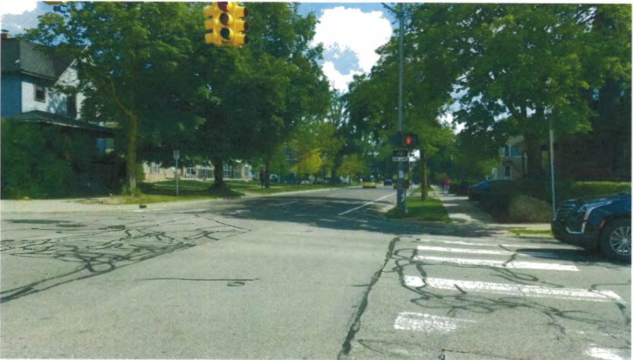
Looking south at Fifth Avenue
