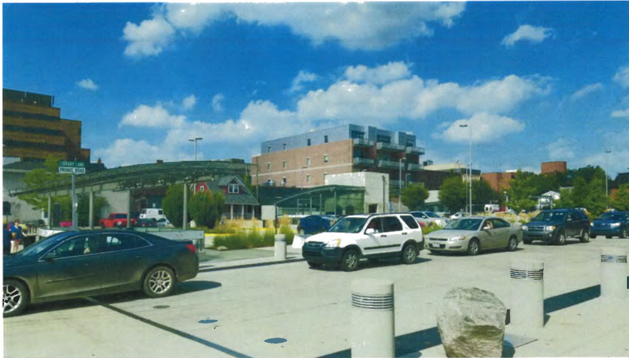
Underground public parking slated for private development above ground contiguous to the north of the public library
