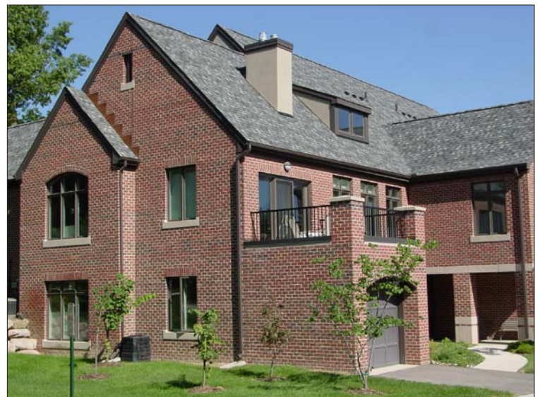
Private residential open space above a garage.
